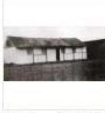
Old Hut and Adjoining Tea Room
